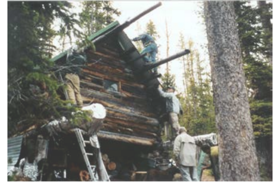
The long over hanging ends were trimmed off
