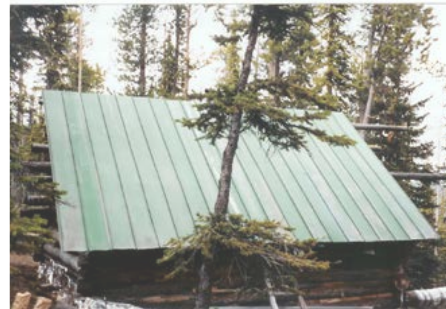
South side finished
