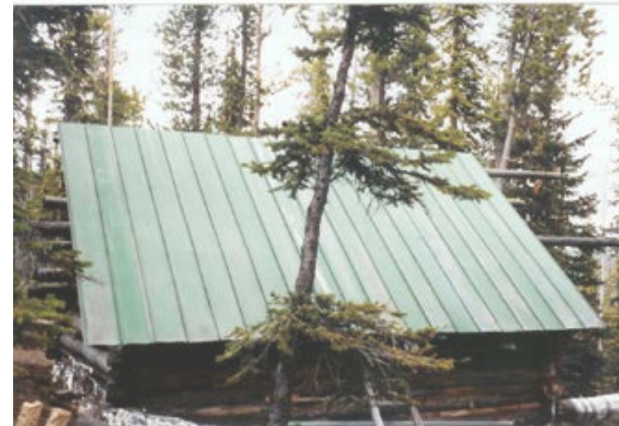
South side finished
