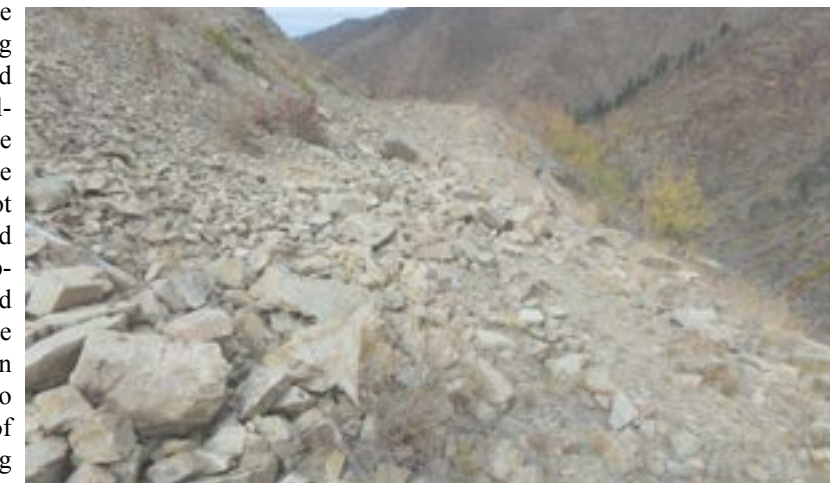
Rockier Section Of The Road
