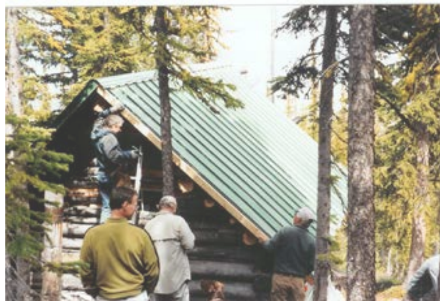
Edges are covered
