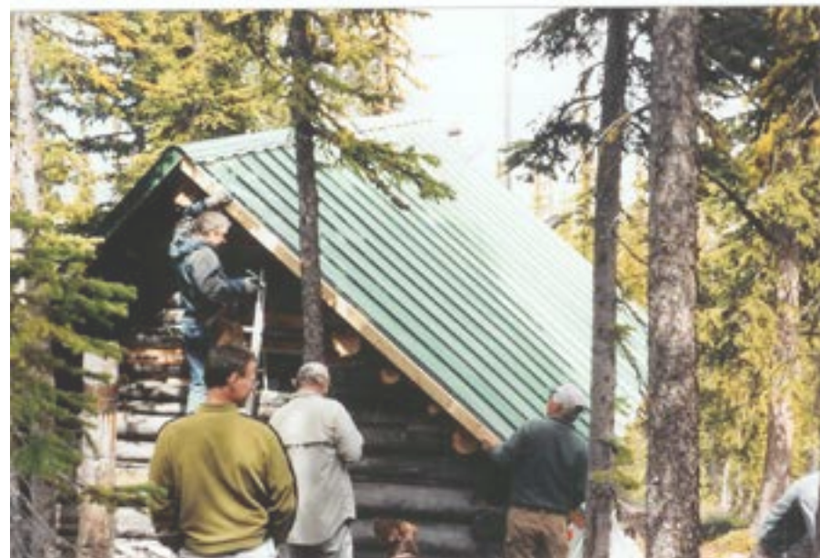
Edges are covered
