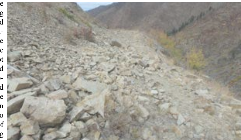
Rockier Section Of The Road
